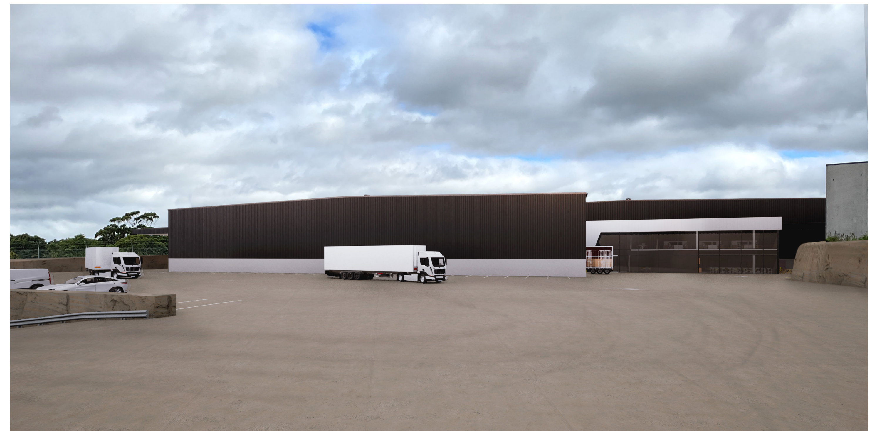
VIEW FROM MAIN ENTRY GATE / PINNACLE PLACE
